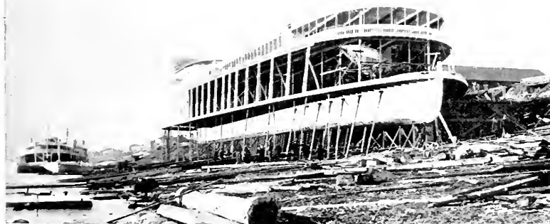
OHIO RIVER PACKET CITY OF LOUISVILLE, 1681 TONS, ON THE STOCKS. Length 301 feet, breadth 42, depth 7.
